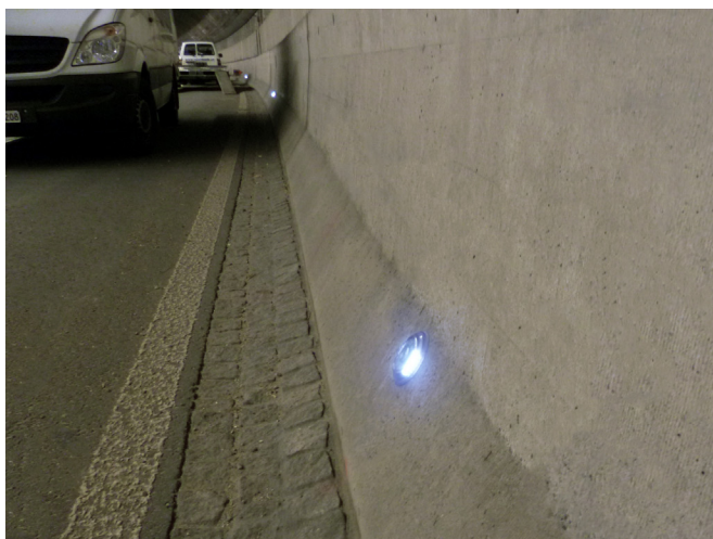
Tunnel Stephanshorn Saint-Gall
